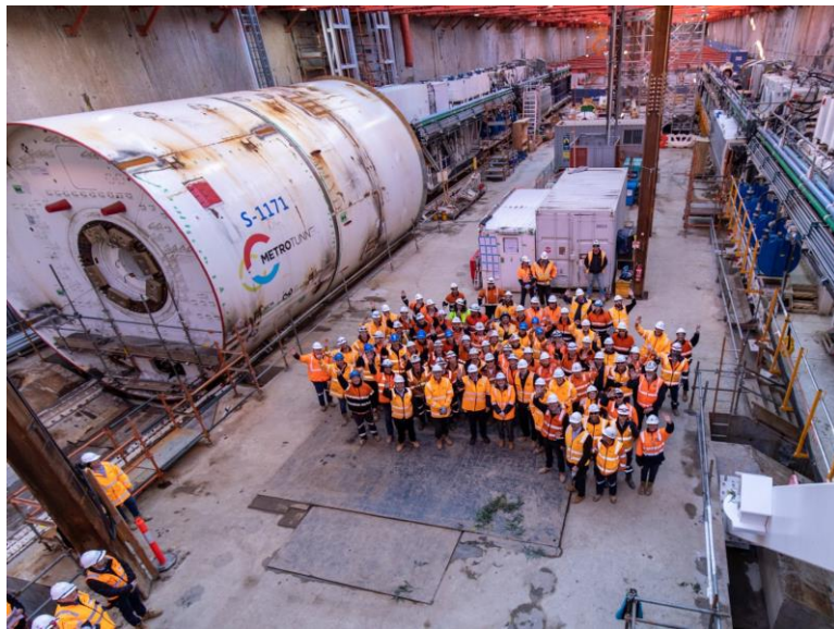
Melbourne Metro – TBM Launch from box shaft (anchored and strutted d-walls)
