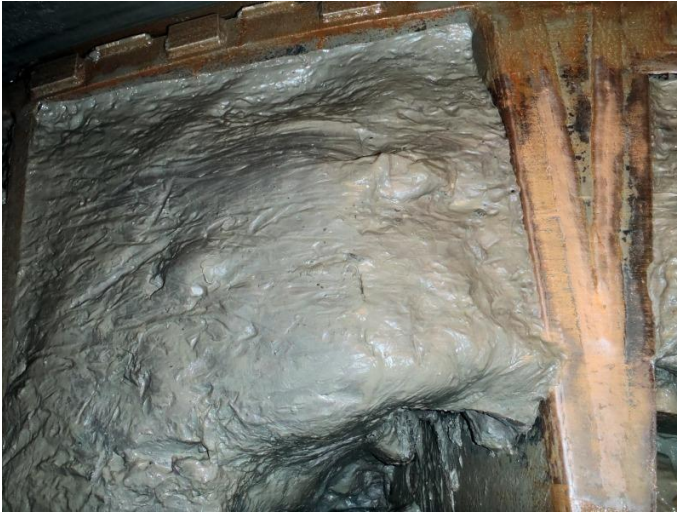
Liefkenshoektunnel – Clogging of the cutterwheel clearly seen – not an Arcadis project
